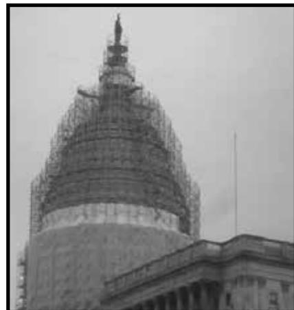
The dome of the U.S. Capitol is made of iron; because of rust and decay, it is currently being restored and repainted.
